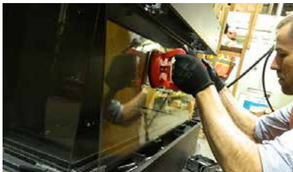
Handle front panel with supplied vacuum clamps
